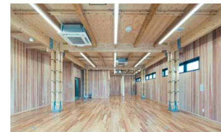
Hospital built using the “Ichu Wood Frame Structure” technique
