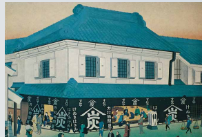
Premises of a Sumiya (a charcoal dealer), from which YUASA TRADING evolved, located in what was formerly the Toriabura-cho neighborhood of the Nihonbashi district of Edo (Tokyo), which is now the Odenma-cho neighborhood of Nihonbashi, and is where YUASA TRADING's head office used to be located.
