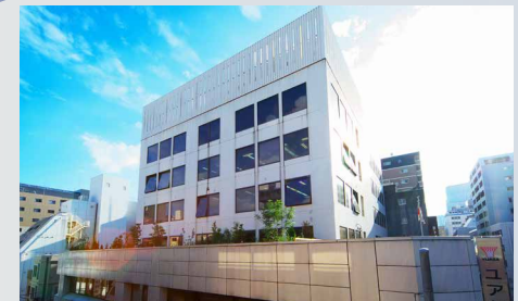
Former head office building in Odenma-cho, Nihonbashi (until 2014)
