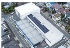
YUASA TRADING Chubu Branch Office (Nagoya, Aichi Prefecture) building
