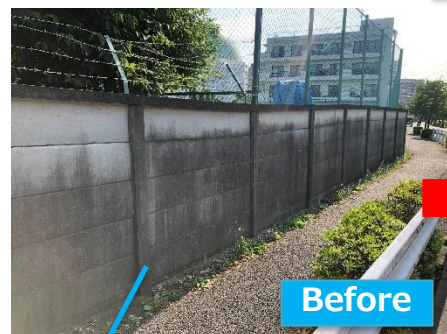
Posts used as they are, no foundation work required
